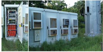
if a power outage occurred at the launch center, the industrial energy storage backup power supply would immediately provide power to the ground control system, ensuring uninterrupted communication for the base.
